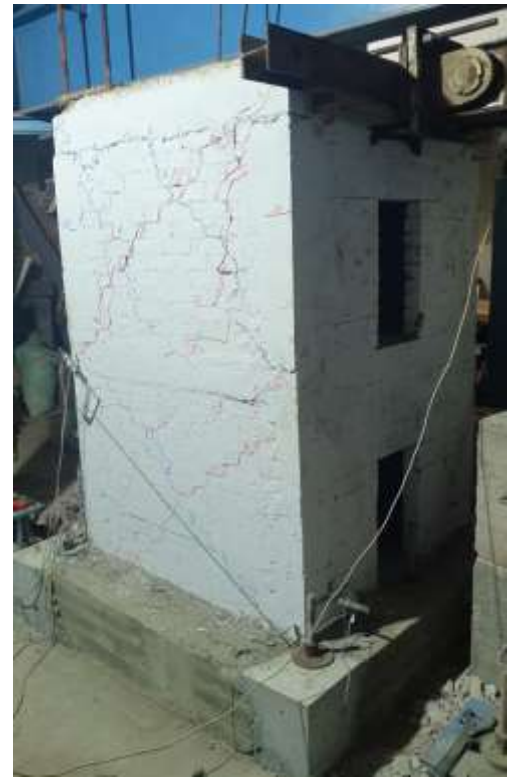
Fig. 12. DS3 Diagonal shear crack
