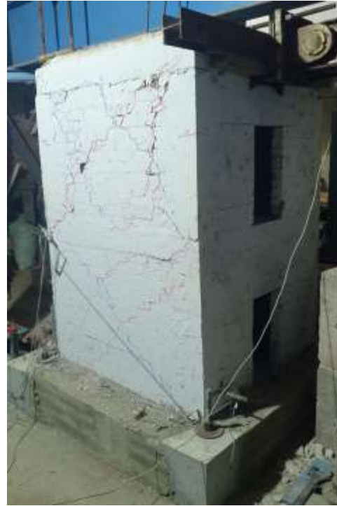
Fig. 14 DS10 Diagonal shear crack at bottom
