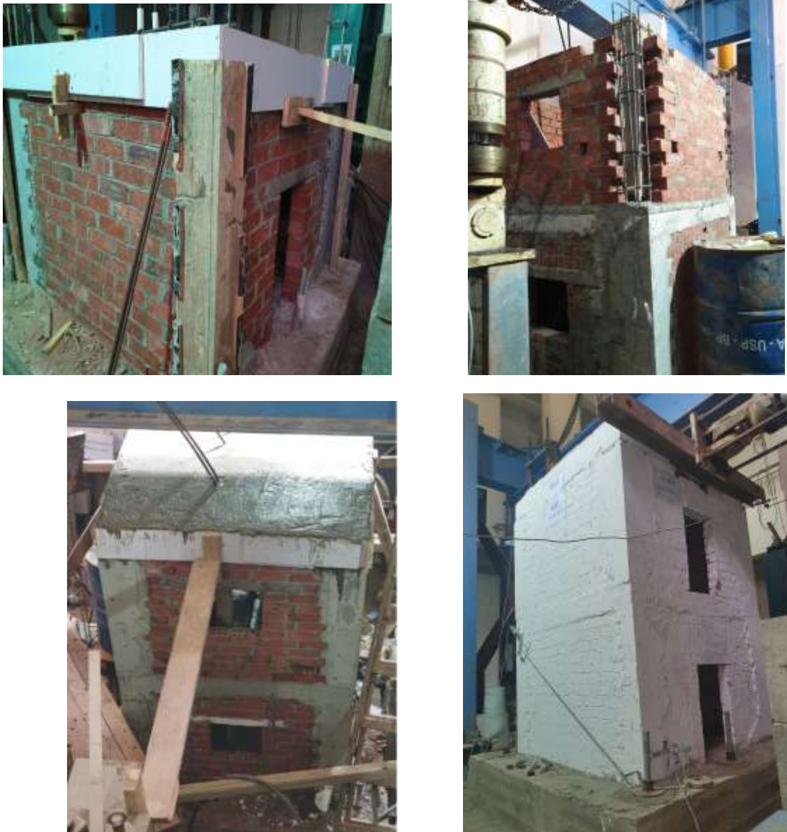
Fig.3. Construction process of specimen.
